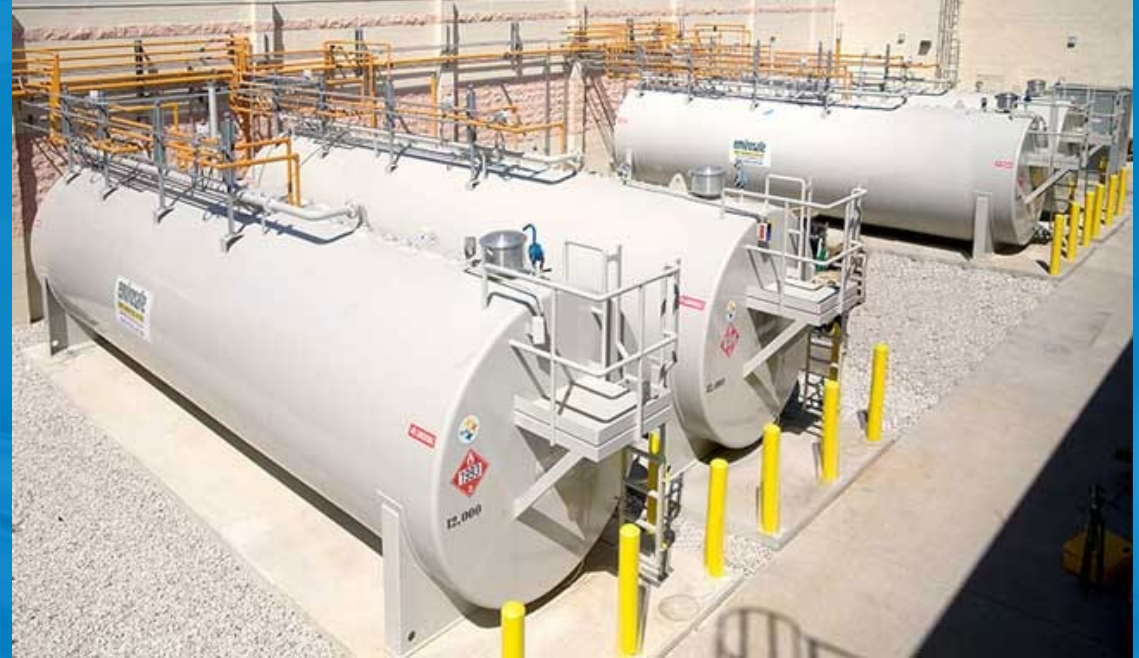
Figure 1. Generator Fuel Storage Tanks
